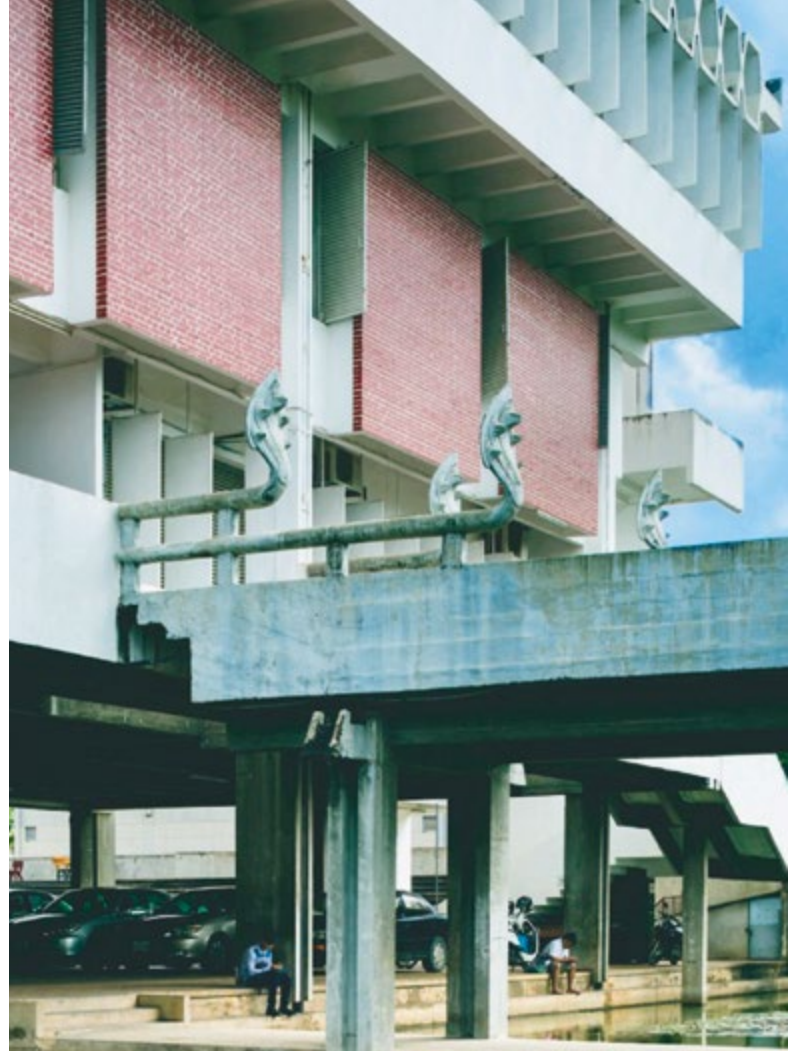
A series of passive strategies adopted by the Architect Vann Molyvann, illustrating the potential of a climate responsive design, protecting buildings from the heat, providing natural air flow and sufficient day lighting, to ensure user thermal comfort. Photo: Shinkenchiku-sha - a+u
