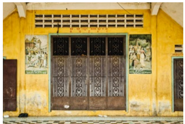
Aerators features on top of building openings, let naturally the hot air escape from the indoor place, helping also to accelerate natural air movement . Photo: Vecteezy.com
