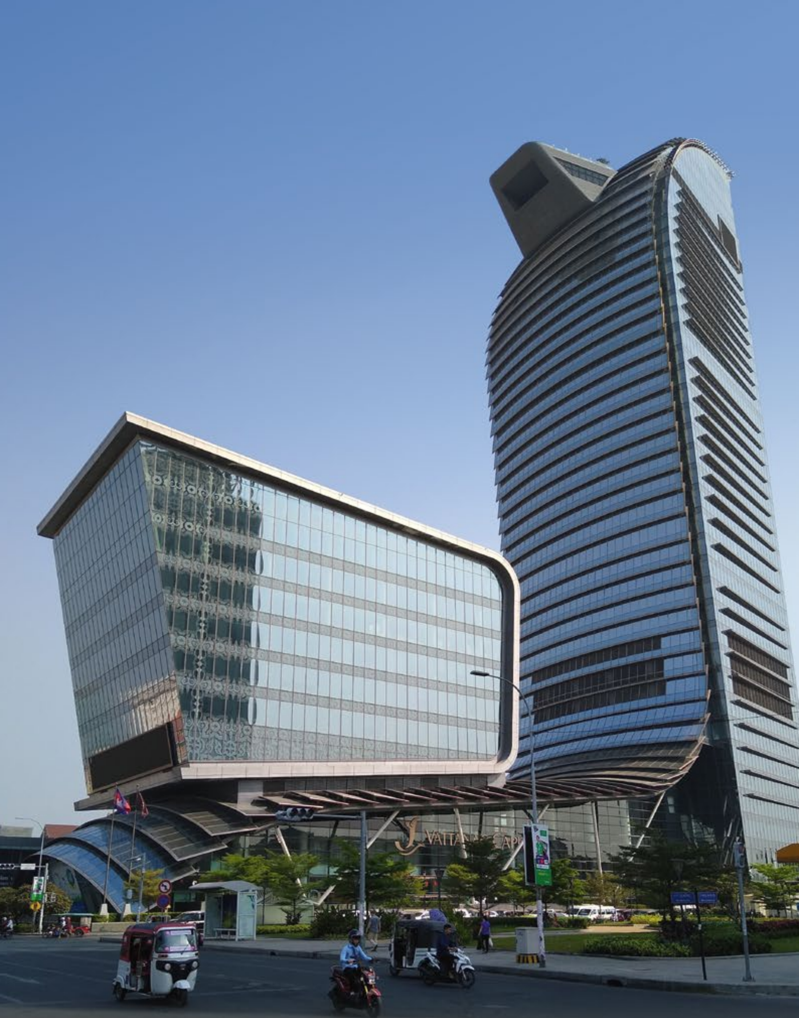
The Vattanac Tower in Phnom Penh, first tower to be Gold LEED green building certified in Cambodia, completed in 2014, with facade shading "scales" among other features. Photo: Wikimedia Commons CC by SA 1.0
