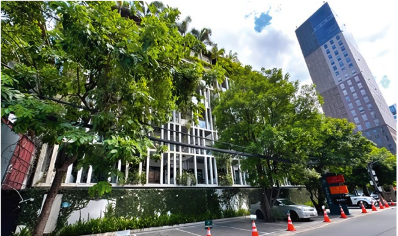
Recessed facade, vertical shading, balconies vegetation, and trees preservation at street level, are keeping the building cooler than surrounding outside ambient air. - Hotel Baitong, Phnom Penh. - Phnom Penh city center. Photo: © A.Cadin & M.Tep.
