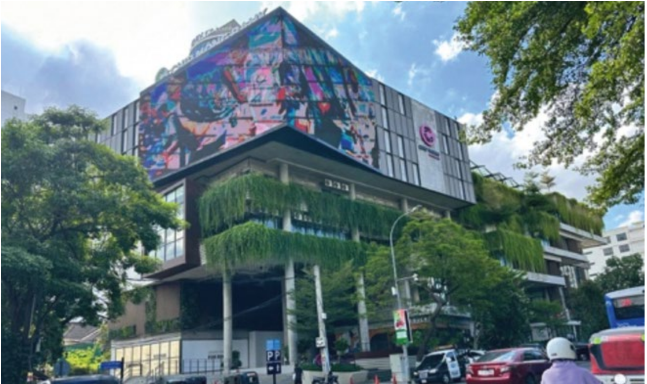
Recent Mixed-use development incorporate passive cooling features such as green walls, waterfalls, and open ventilation, creating more attractive spaces for people within and around these innovative structures. Photo: © A.Cadin & M.Tep.
