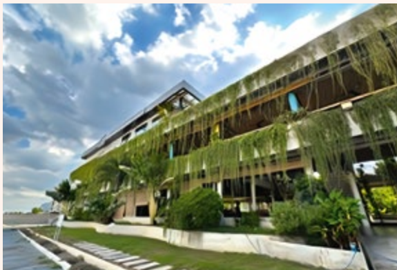
Local trends of sustainable design are integrating open common areas with natural ventilation and building green facades. Photo: A.Cadin & M.Tep
