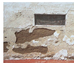
Figure 82: Peeling of exterior wall
