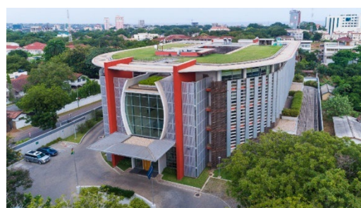
Figure 88: Green roof on building of World Bank Group Office, Accra, Ghana
