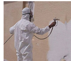
Figure 84: Spraying of final coat surfaces for
