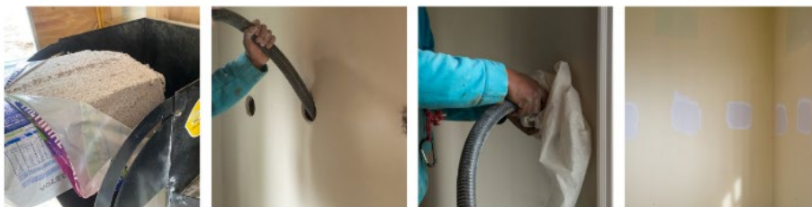
Figure 74 Cellulose Insulation Installation
