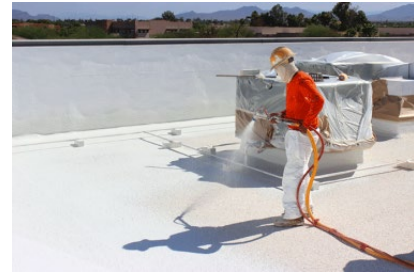
Figure 95: Roof coating
