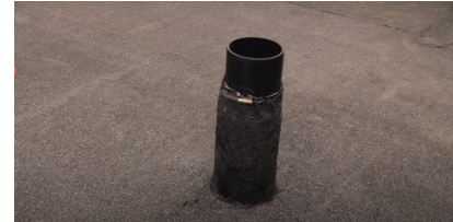
Figure 96: Installation of modified bitumen
